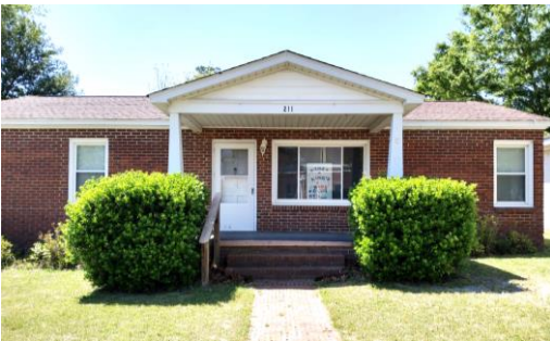
The "Staff House" new location
